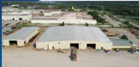
Sand Springs, OK | Bundle Fabrication
