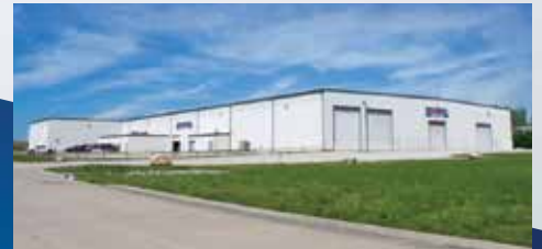
Catoosa, OK | ACHE & Structural Steel Fabrication
