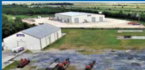
Beaumont, TX | Fabrication
