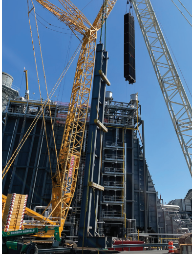
HP Economizer Coil Replacement
