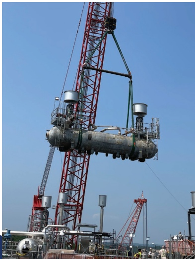
Steam Drum Removal
