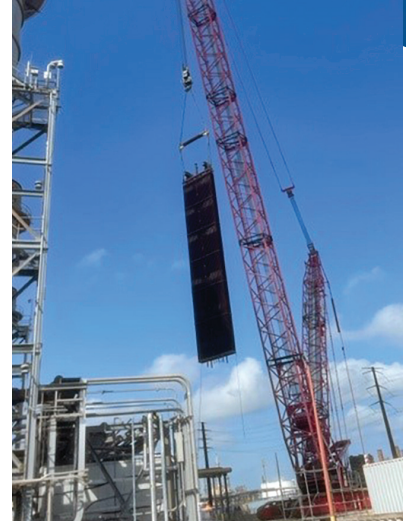
Economizer Module Replacement
