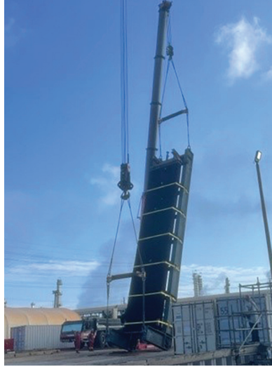
Economizer Coil Replacement
