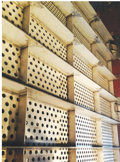
Flow Grid Installation
